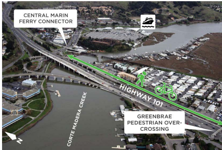
The environmentally sound alignment for the North-South Ferry Connector Path
